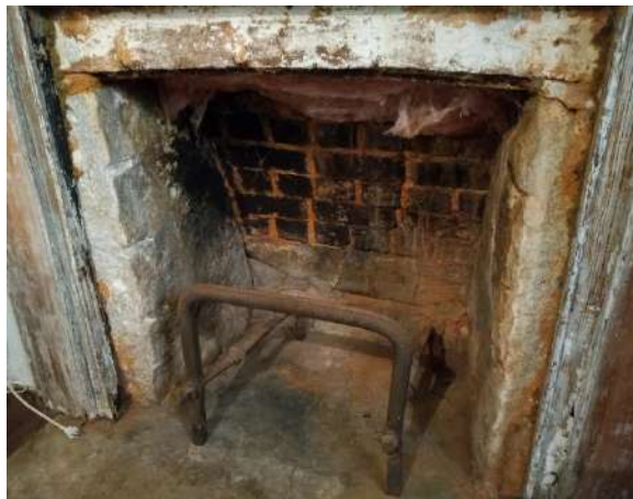
This photo is from another house in Oakway built by the same builders in late 1800s. The fireplaces are all of the exact same style: solid rock sides and brick starting from the middle of the firebox and up.
