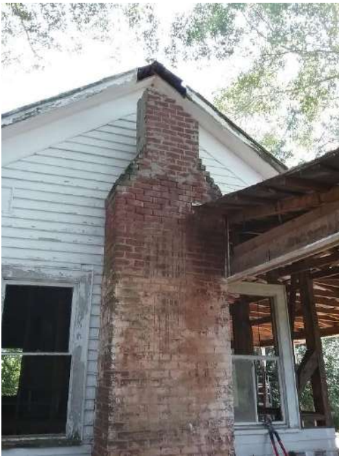
Photo of 1 (of 3) chimneys to be rebuilt. This photo was taken shortly after the dismantling began.
